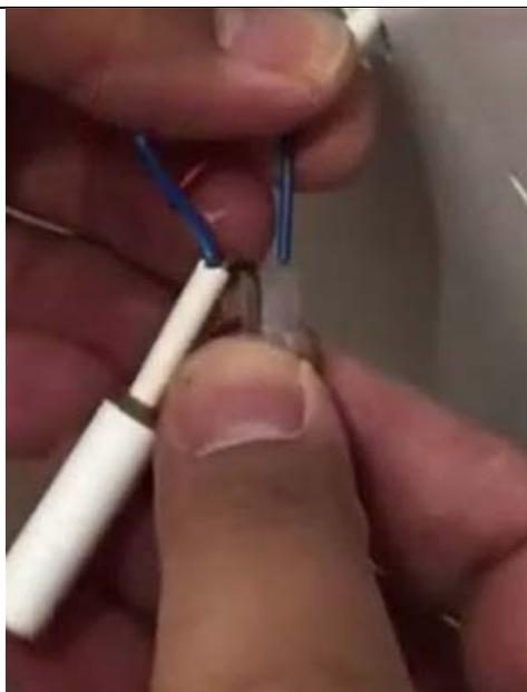
3. Join the old and new temperature sensor cables using the scotchlok
